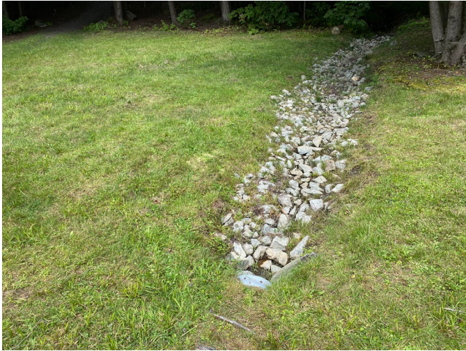
Existing dry swale (rock lined swale)
