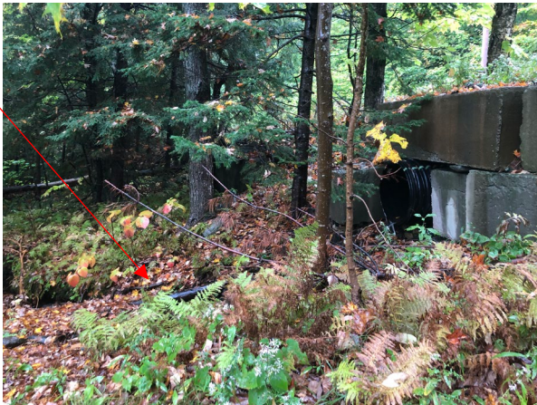
Existing plunge pool, debris build up on left of picture, to be removed
