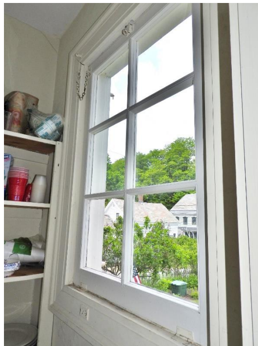
Window 1. This hopper window is in good condition, with areas of peeling paint, and the exterior glazing may need replacement.
