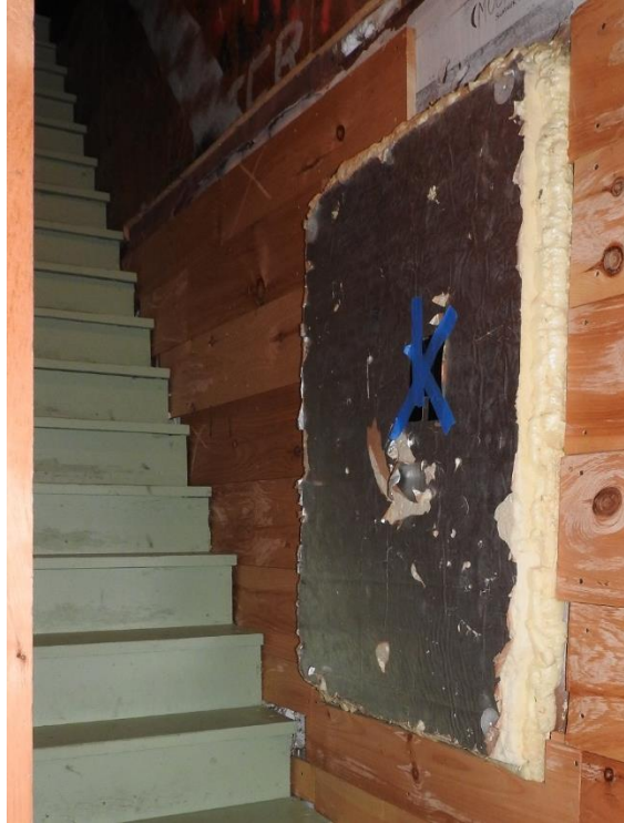
Window 12. This hopper window has areas of peeling paint, has been fixed closed, and the exterior glazing may need replacement. It is blocked on the interior with insulation.
