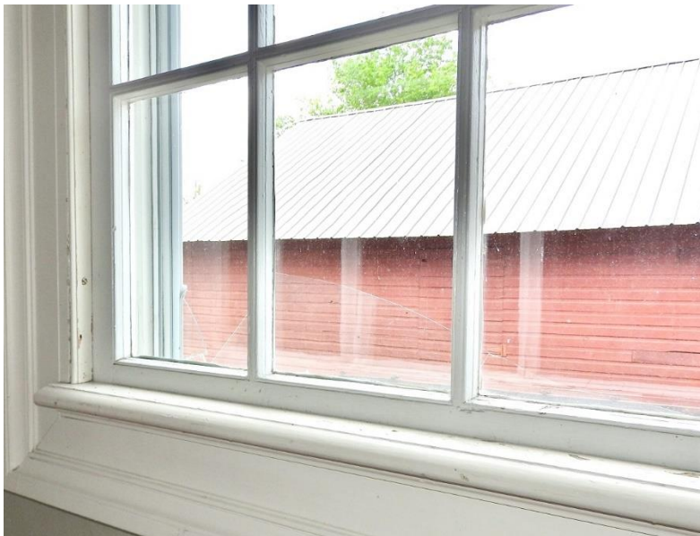
Window 19. This double-hung window is in good condition, with areas of peeling paint, and the exterior glazing may need replacement. Note how the meeting rails of the wood windows and storm window do not align, and one storm sash is broken.
