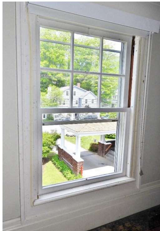
Window 3. This double-hung window is in good condition, with areas of peeling paint, and the exterior glazing may need replacement. One sash of the storm window is missing.
