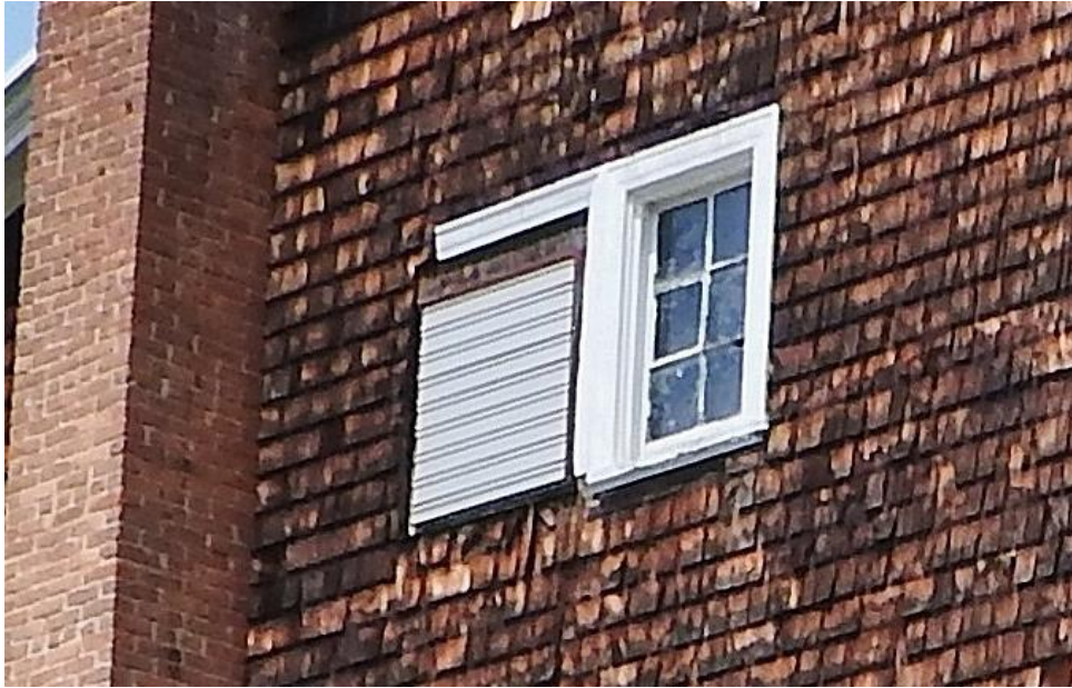
Window 39. This was originally a paired window. The remaining sash is in poor condition.
