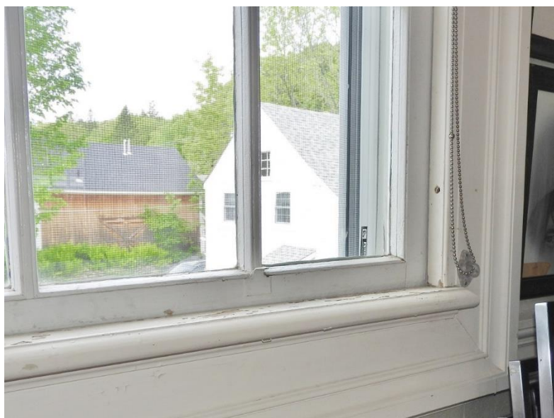
Window 16. This double-hung window with fanlight is in good condition, with areas of peeling paint, and the exterior glazing may need replacement. Note how the meeting rails of the wood windows and storm window do not align.
