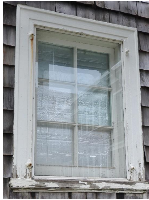
Windows 22 and 23. These hopper windows have areas of peeling paint, have been fixed closed, and the exterior glazing may need replacement. They are blocked on the interior with insulation.
