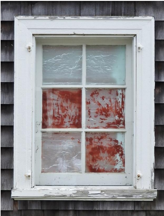
Windows 10 and 11. These hopper windows have areas of peeling paint, have been fixed closed, and the exterior glazing may need replacement. They are blocked on the interior with insulation.
