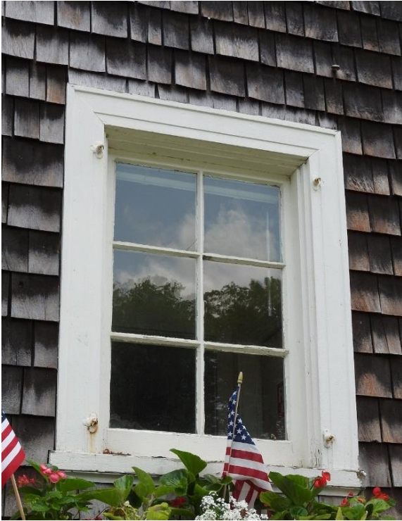
Window 2. This hopper window is in good condition, with areas of peeling paint, and the exterior glazing may need replacement.
