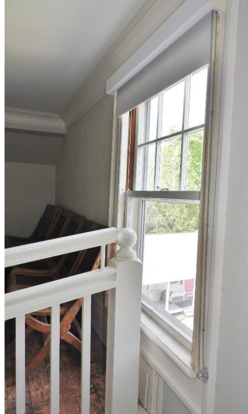
Window 5. This double-hung window is in good condition, with areas of peeling paint, and the exterior glazing may need replacement.
