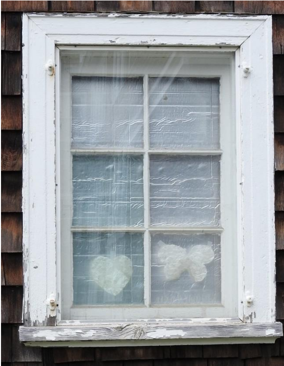
Window 24. This hopper window has areas of peeling paint, has been fixed closed, and the exterior glazing may need replacement. It is blocked on the interior with insulation.
