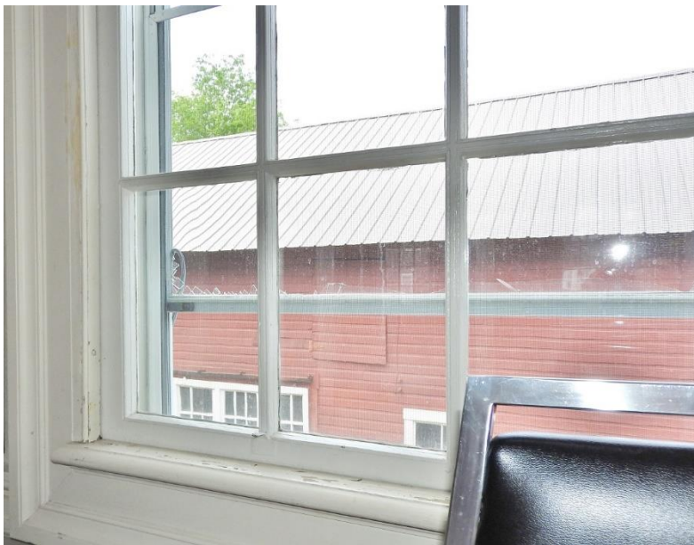
Window 18. This double-hung window with fanlight is in good condition, with areas of peeling paint, and the exterior glazing may need replacement. Note how the meeting rails of the wood windows and storm window do not align, and one storm sash is broken.
