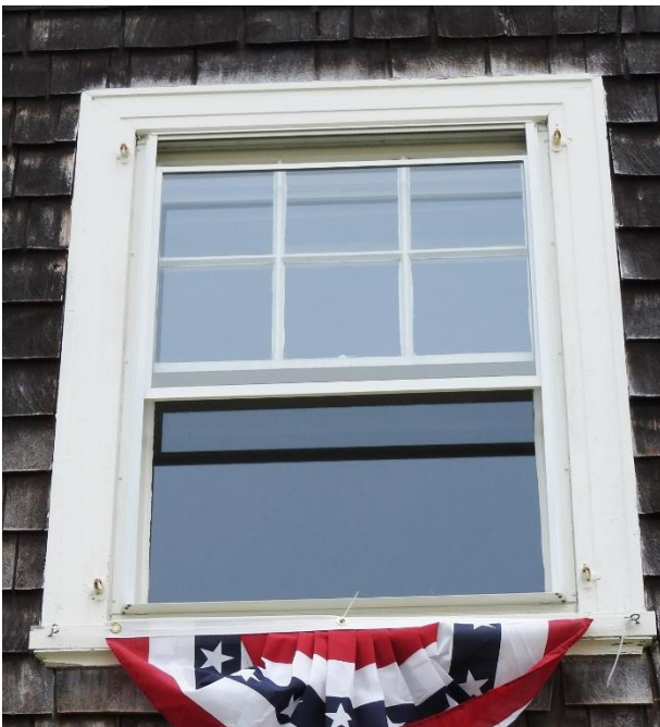
Window 2. This hopper window is in good condition, with areas of peeling paint, and the exterior glazing may need replacement.
