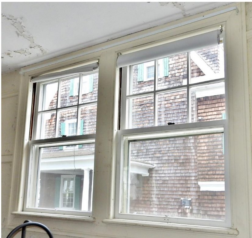
Windows 32 and 33. These double-hung windows are in good condition, have areas of peeling paint, and the exterior glazing may need replacement.
