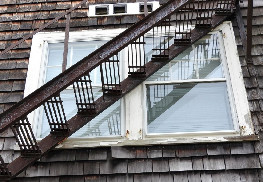
Windows 13 and 14. These double-hung windows are in good condition, have areas of peeling paint, and the exterior glazing may need replacement.
