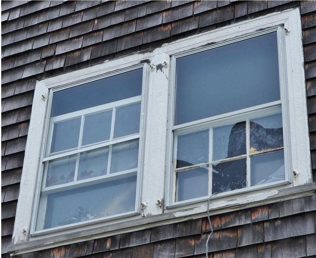
Windows 20 and 21. These double-hung windows are not properly closed, have deteriorated glazing, and broken storm sash. They are blocked on the interior.
