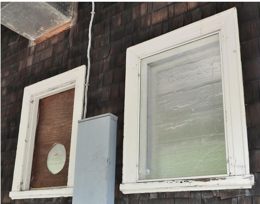
Windows 34, 35, 36, 37 and 38. These basement windows are in good condition, with areas of peeling paint. The glass pane of Window 37 has been removed. All of the windows are blocked on the interior with insulation.
