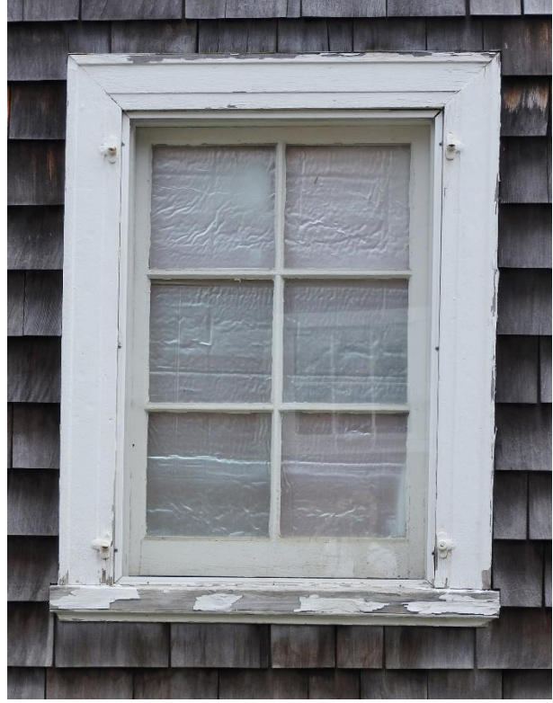
Windows 8 and 9. These hopper windows have areas of peeling paint, have been fixed closed, and the exterior glazing may need replacement. They are blocked on the interior with insulation.
