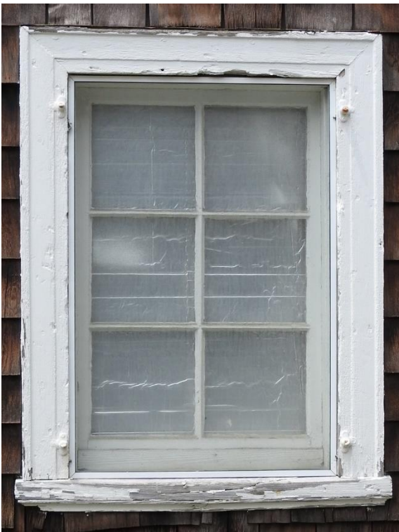
Windows 25 and 26. These hopper windows have areas of peeling paint, have been fixed closed, and the exterior glazing may need replacement. They are blocked on the interior with insulation.
