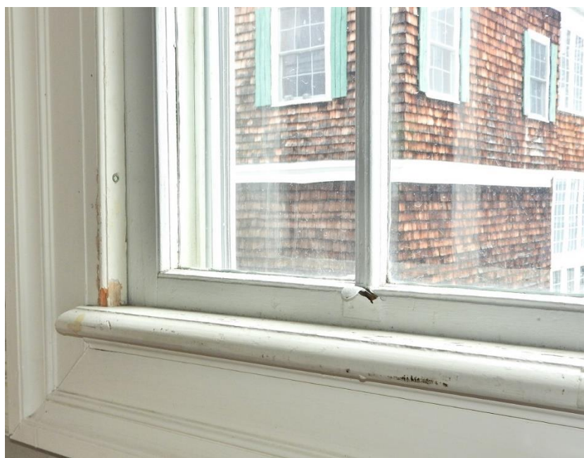
Window 28. This double-hung window with fanlight is in good condition, with areas of peeling paint, and the exterior glazing may need replacement. On this side of the building, the meeting rails of the storm sash align with the wood windows, but some sash are out of alignment and there is loose weather stripping.
