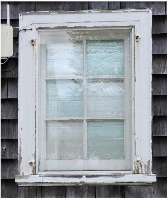
Windows 6 and 7. These hopper windows have areas of peeling paint, have been fixed closed, and the exterior glazing may need replacement. They are blocked on the interior with insulation.
