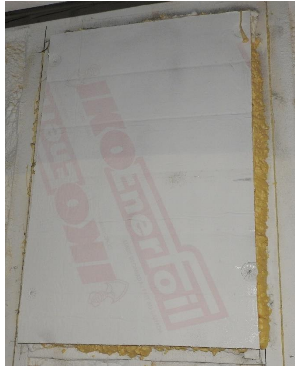
Window 24. This hopper window has areas of peeling paint, has been fixed closed, and the exterior glazing may need replacement. It is blocked on the interior with insulation.
