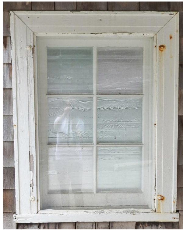
Windows 25 and 26. These hopper windows have areas of peeling paint, have been fixed closed, and the exterior glazing may need replacement. They are blocked on the interior with insulation.
