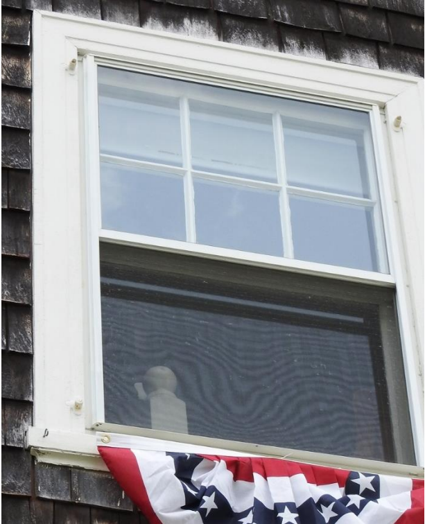
Window 5. This double-hung window is in good condition, with areas of peeling paint, and the exterior glazing may need replacement.
