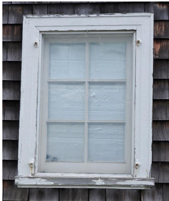
Windows 6 and 7. These hopper windows have areas of peeling paint, have been fixed closed, and the exterior glazing may need replacement. They are blocked on the interior with insulation.
