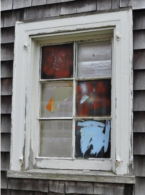
Window 12. This hopper window has areas of peeling paint, has been fixed closed, and the exterior glazing may need replacement. It is blocked on the interior with insulation.
