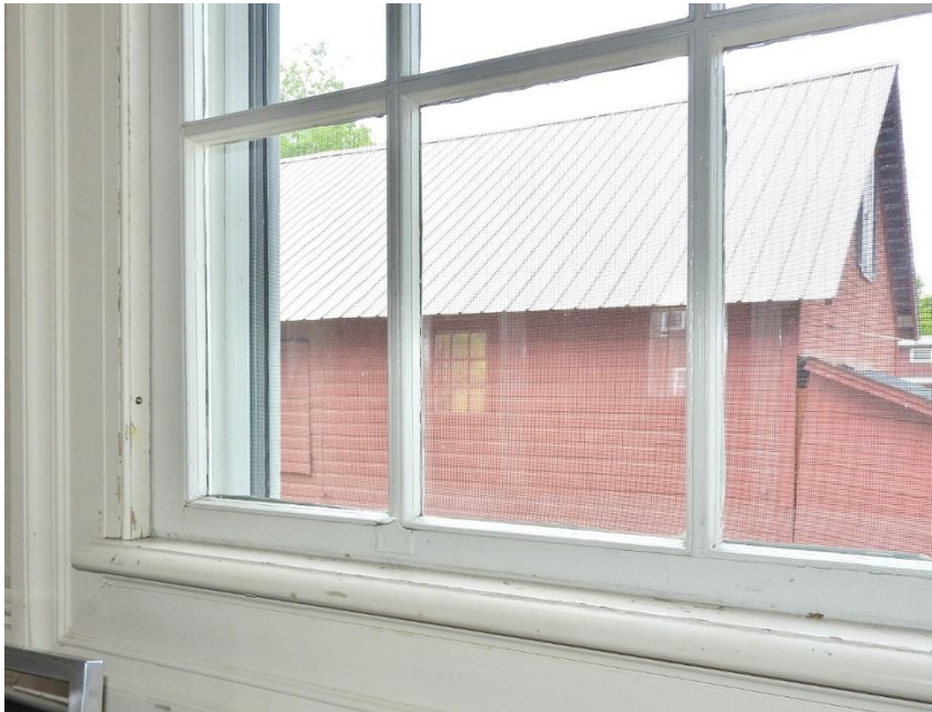
Window 17. This double-hung window with fanlight is in good condition, with areas of peeling paint, and the exterior glazing may need replacement. Note how the meeting rails of the wood windows and storm window do not align.
