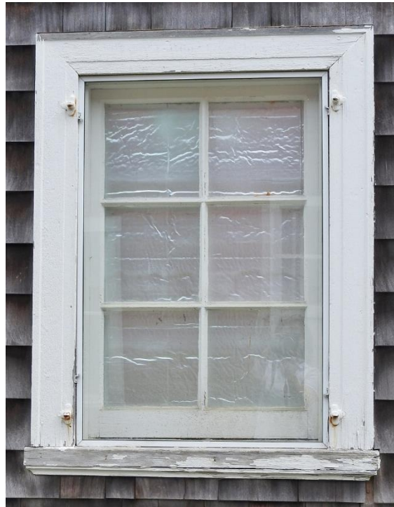
Windows 10 and 11. These hopper windows have areas of peeling paint, have been fixed closed, and the exterior glazing may need replacement. They are blocked on the interior with insulation.
