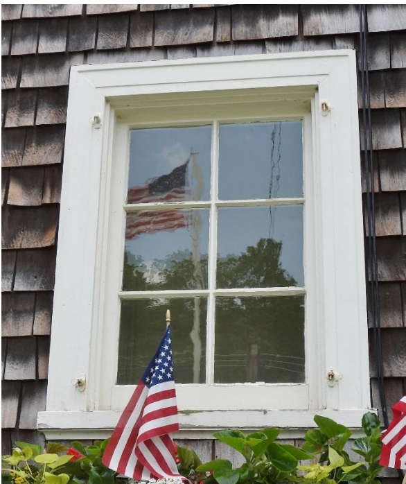
Window 1. This hopper window is in good condition, with areas of peeling paint, and the exterior glazing may need replacement.
