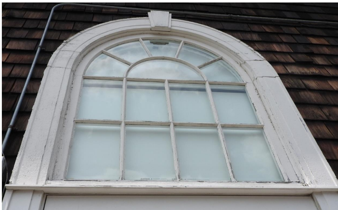
Window 31. This window and fanlight surmount a door. They are in good condition, with areas of peeling paint, and the exterior glazing needs replacement.
