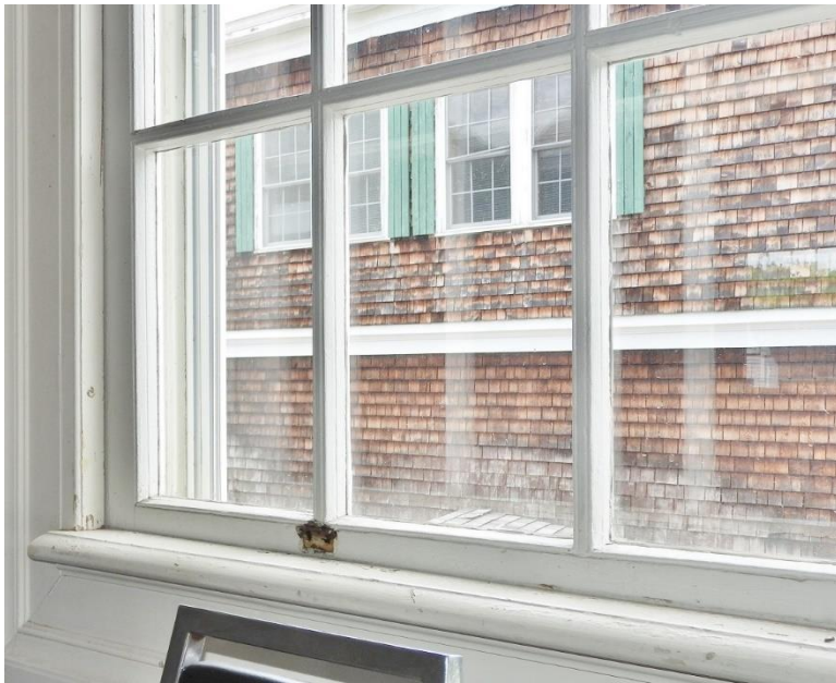
Window 30. This double-hung window with fanlight is in good condition, with areas of peeling paint, and the exterior glazing may need replacement. On this side of the building, the meeting rails of the storm sash align with the wood windows, but some sash are out of alignment and there is loose weather stripping.
