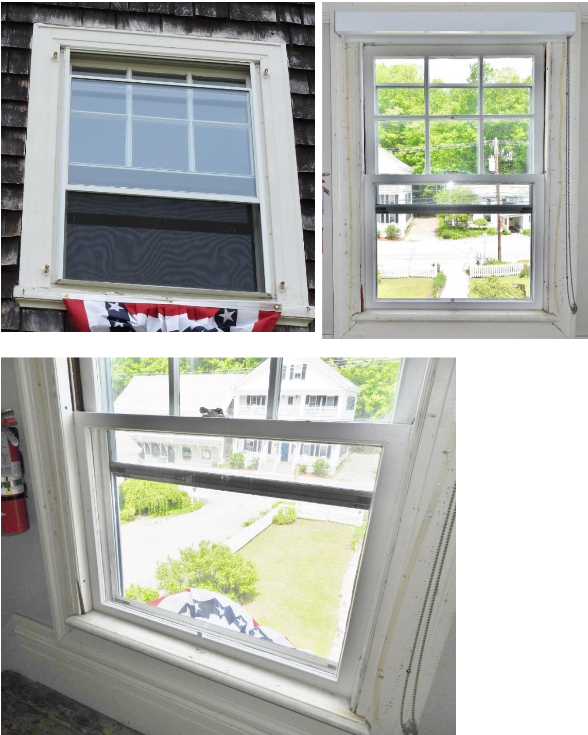
Window 4. This double-hung window is in good condition, with areas of peeling paint, and the exterior glazing may need replacement.
