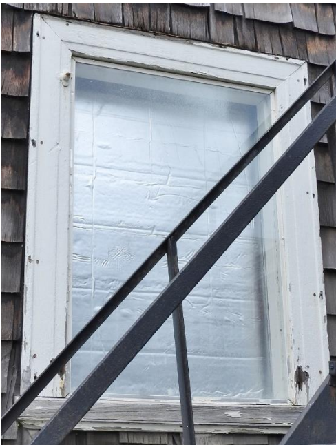
Windows 22 and 23. These hopper windows have areas of peeling paint, have been fixed closed, and the exterior glazing may need replacement. They are blocked on the interior with insulation.
