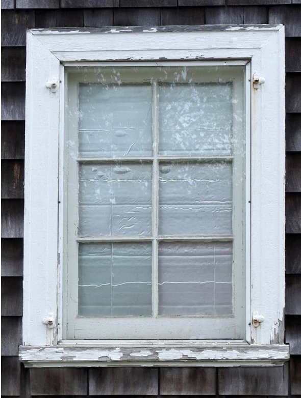
Windows 8 and 9. These hopper windows have areas of peeling paint, have been fixed closed, and the exterior glazing may need replacement. They are blocked on the interior with insulation.
