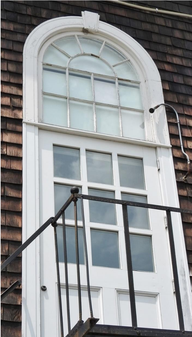
Window 27. This window and fanlight surmount a door. They are in good condition, with areas of peeling paint, and the exterior glazing may need replacement.
