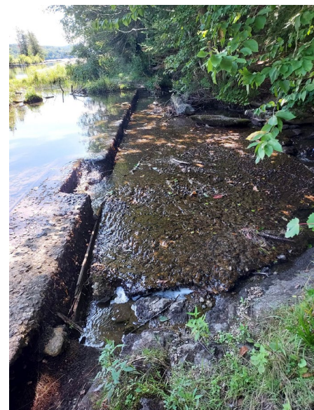
Broad crested spillway looking south
