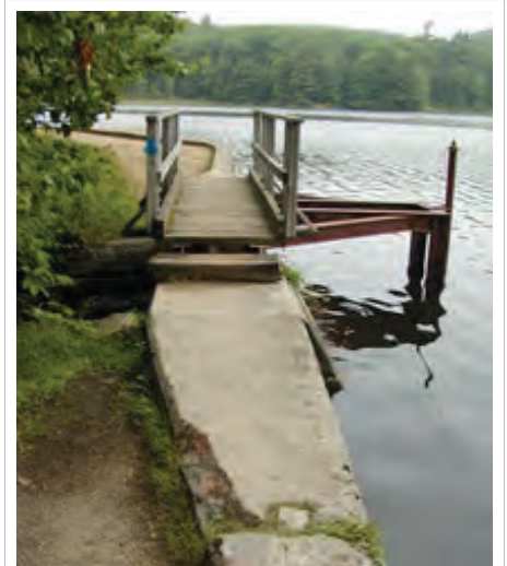
Existing spillway, bridge, and low level outlet gate operator
