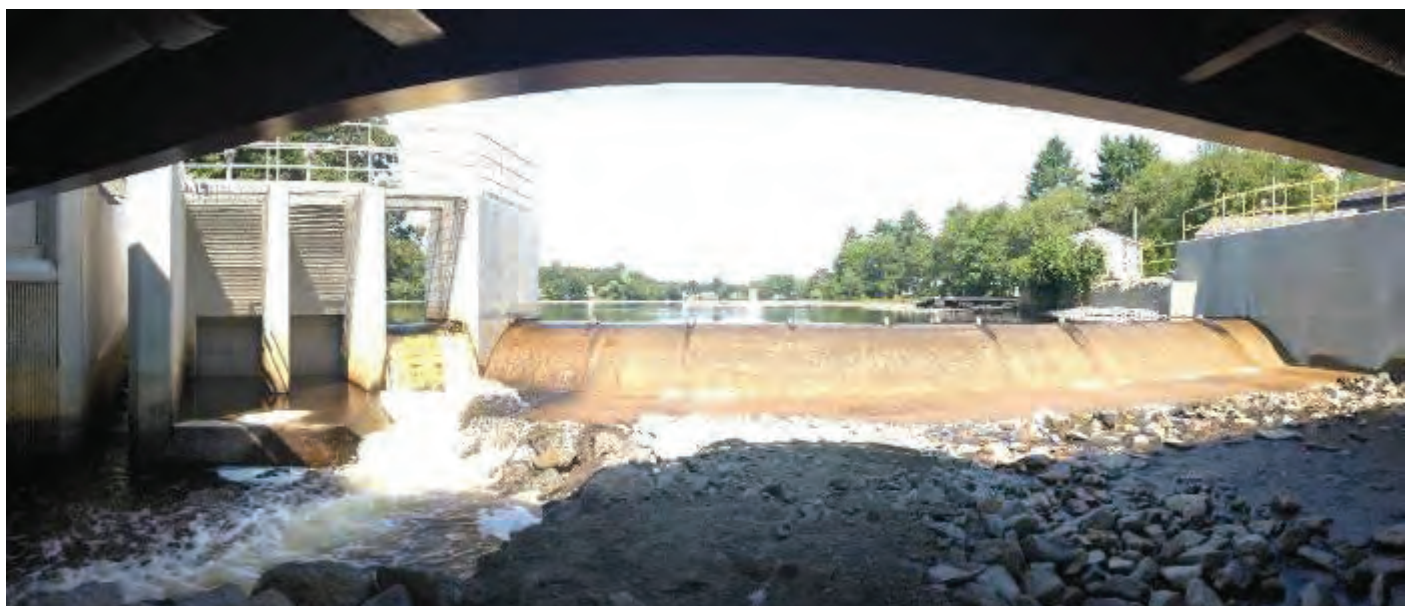
From left to right: Reconstructed fish ladder, outlet gates, stoplog bay, and reinforced concrete ogee spillway
