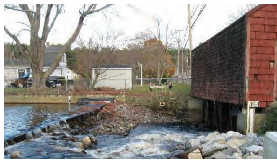
Previous overflow weir (left) and gate structure (right) before replacement
