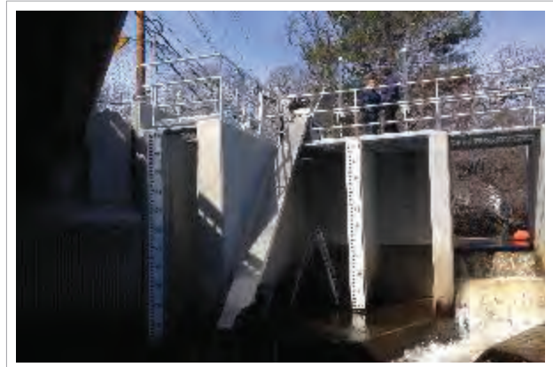
Outlet structure with seasonal eel ladder in place (center)
