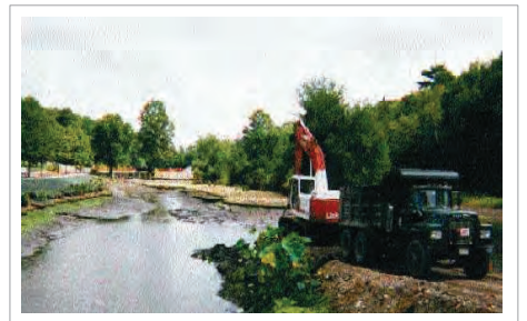
Excavation of sediments using conventional methods
