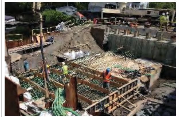
Spillway reinforcement (foreground) and secant pile training wall (background)
