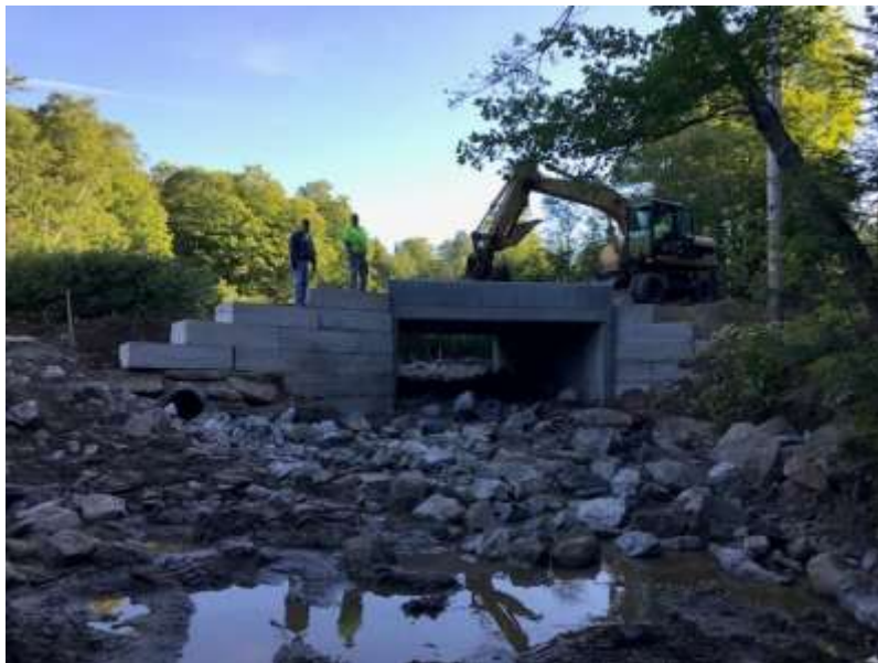
Road crew working on the Ballou Hill culvert replacement
