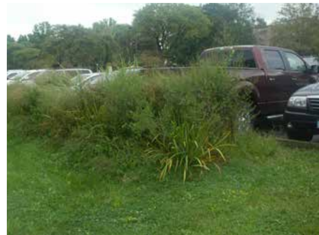
A rain garden installed in a parking lot stores and infiltrates stormwater. Overflow basins, elevated nine to twelve inches above the lowest point in the rain garden, may be installed to divert water during large storm events.
